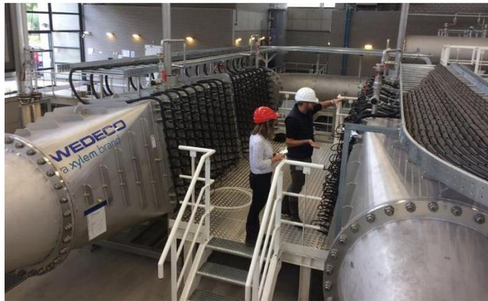
eventually led to the implementation of a full scale research system with a treatment capacity of 2,200 m<sup>3</sup>/hr in 2016. It is currently undergoing final performance tests, and according to Dunea, will represent the first full-scale system using sequential AOP for potable water treatment in the world. The technology has been commercialised by Xylem and is now known as *MiPRO eco3 plus*.
